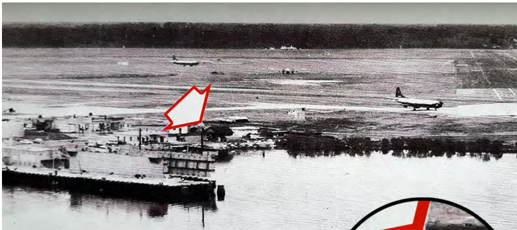
The 43-foot I-beam extended 16.6 feet into the 50/1 approach slope.
