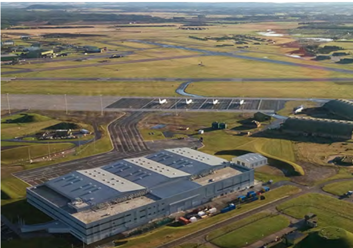
The Atlantic Building and Poseidon Parking Ramp at RAF Lossiemouth.
