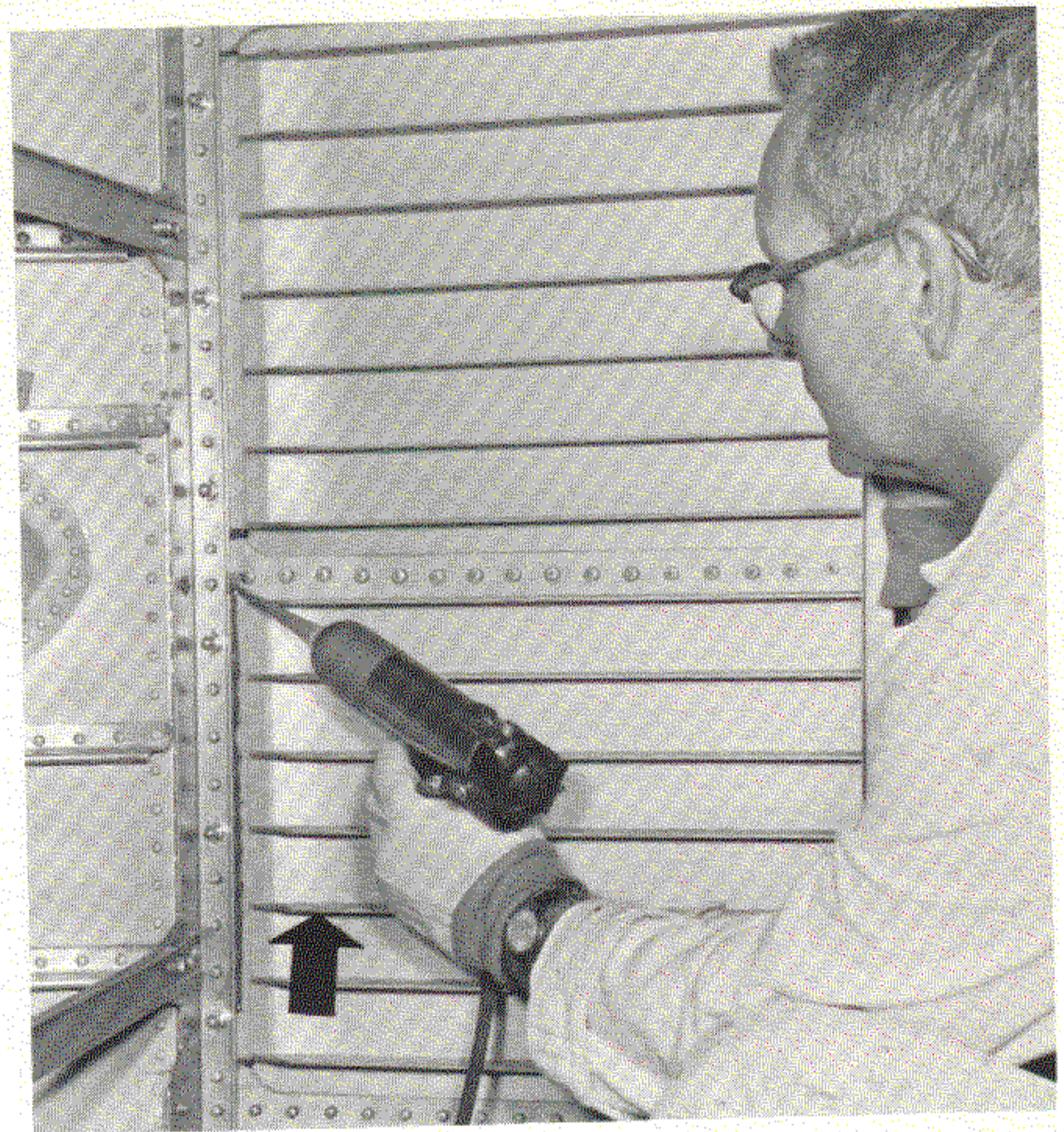
Figure 7 Application of Filleting Compound with Gun
