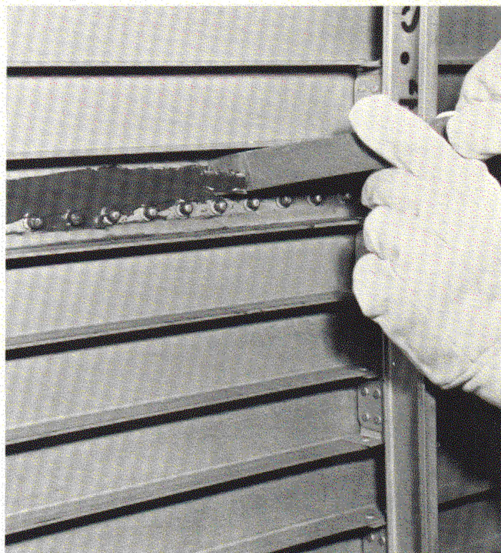
Figure 13 Removing Defective Sealant
