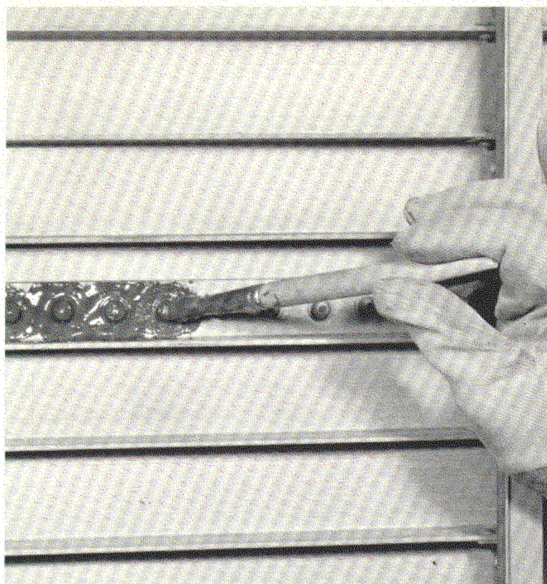
Figure 8 Brush Sealing over Fasteners
