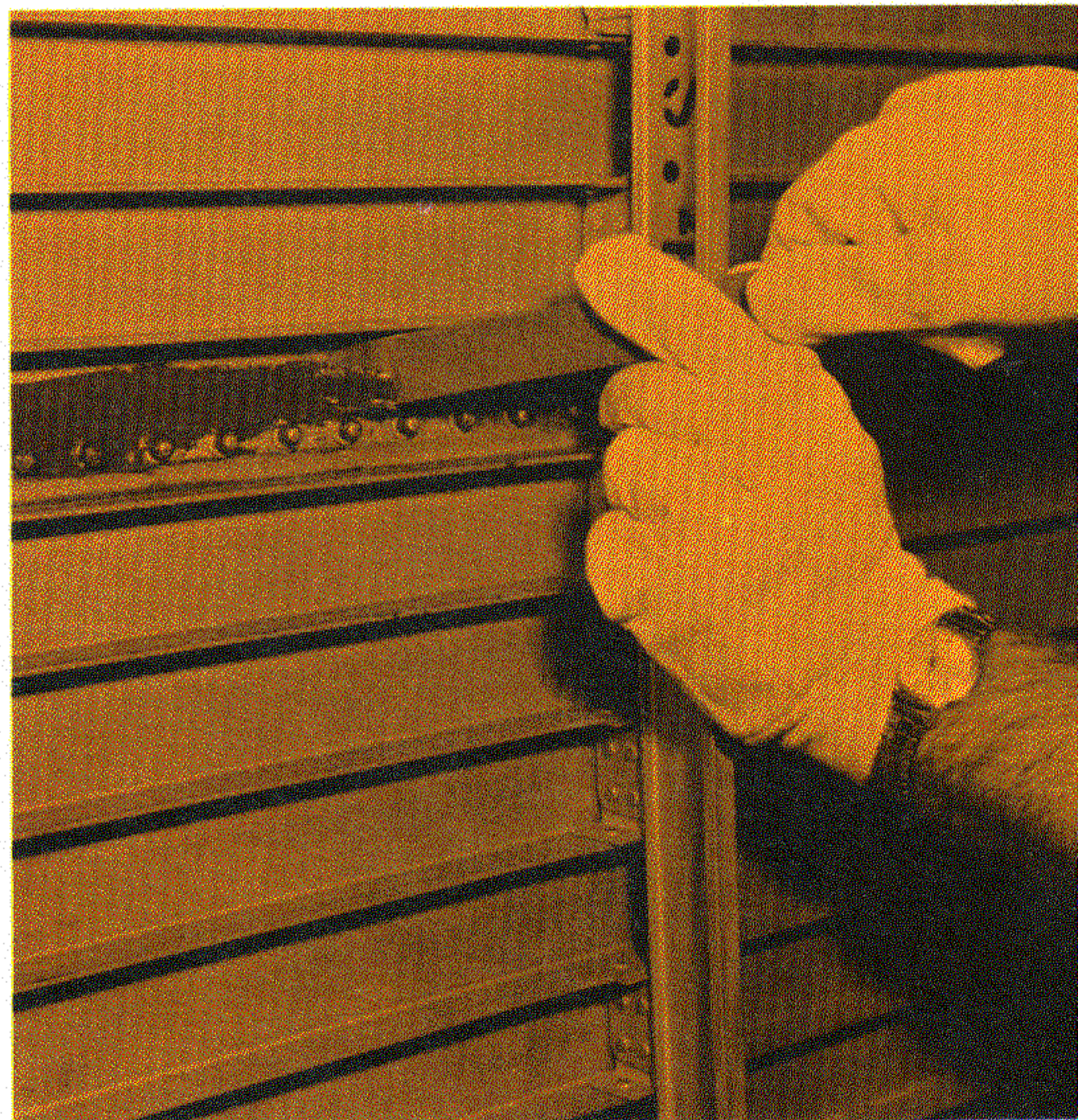
Figure 21. Removing Defective Sealant
