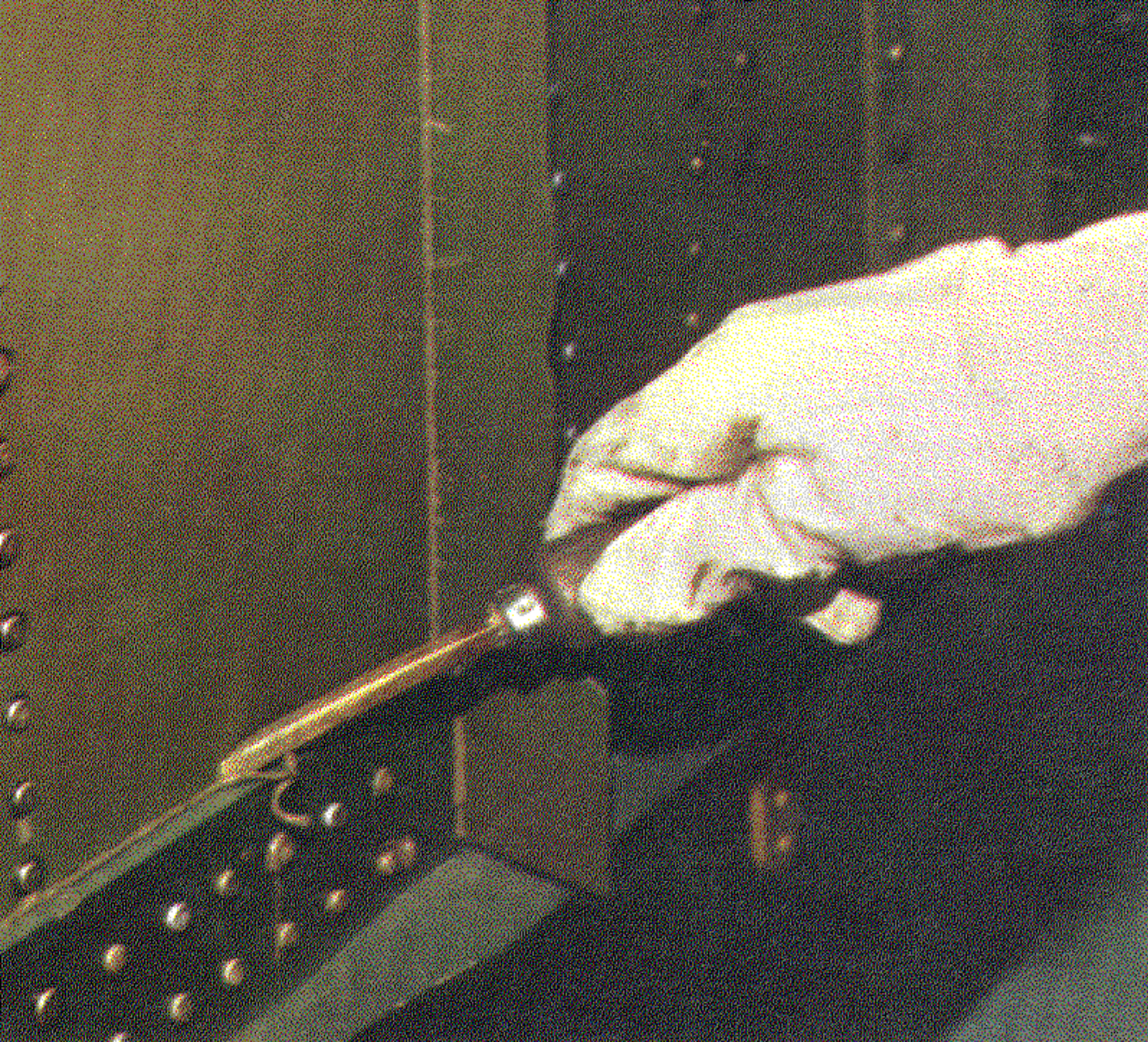
Figure 9. Excessive Sealant is Removed with a Scraper
