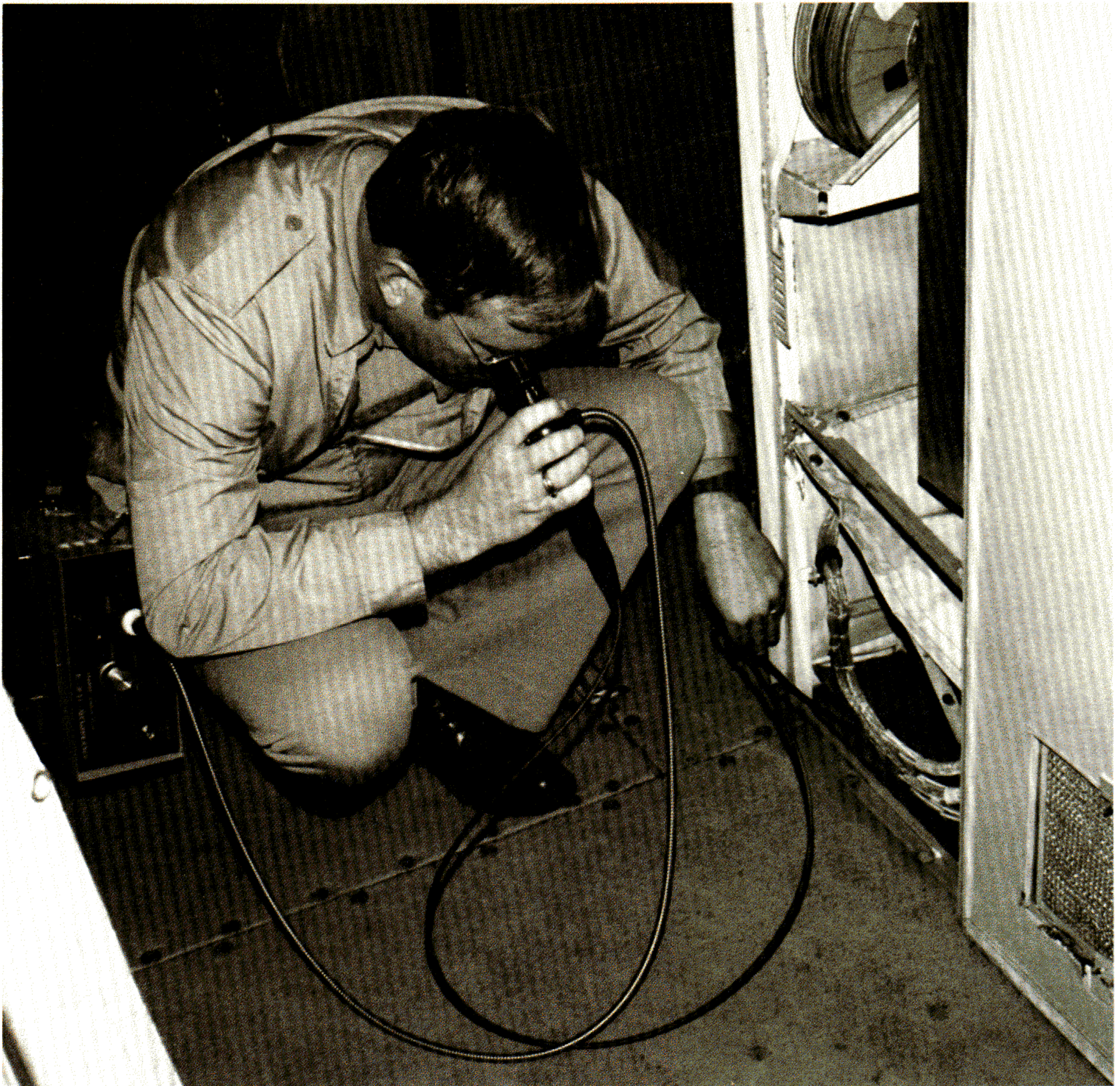
Figure 16. Maintenance Technician Using Fiberoptic Borescope to Inspect Areas Beneath an Electronics Rack.
